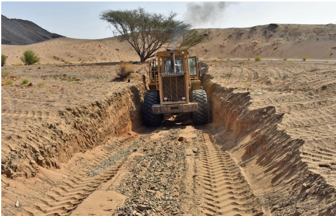
Fig 18. Excavating in alluvial sediments, Romeit area.
