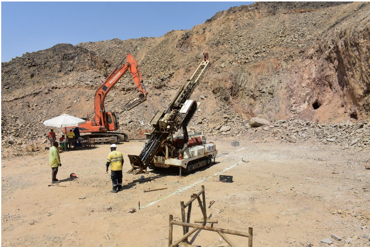
Figure 19. Set up of Diamond Drilling equipment for drill hole RMDD003.
