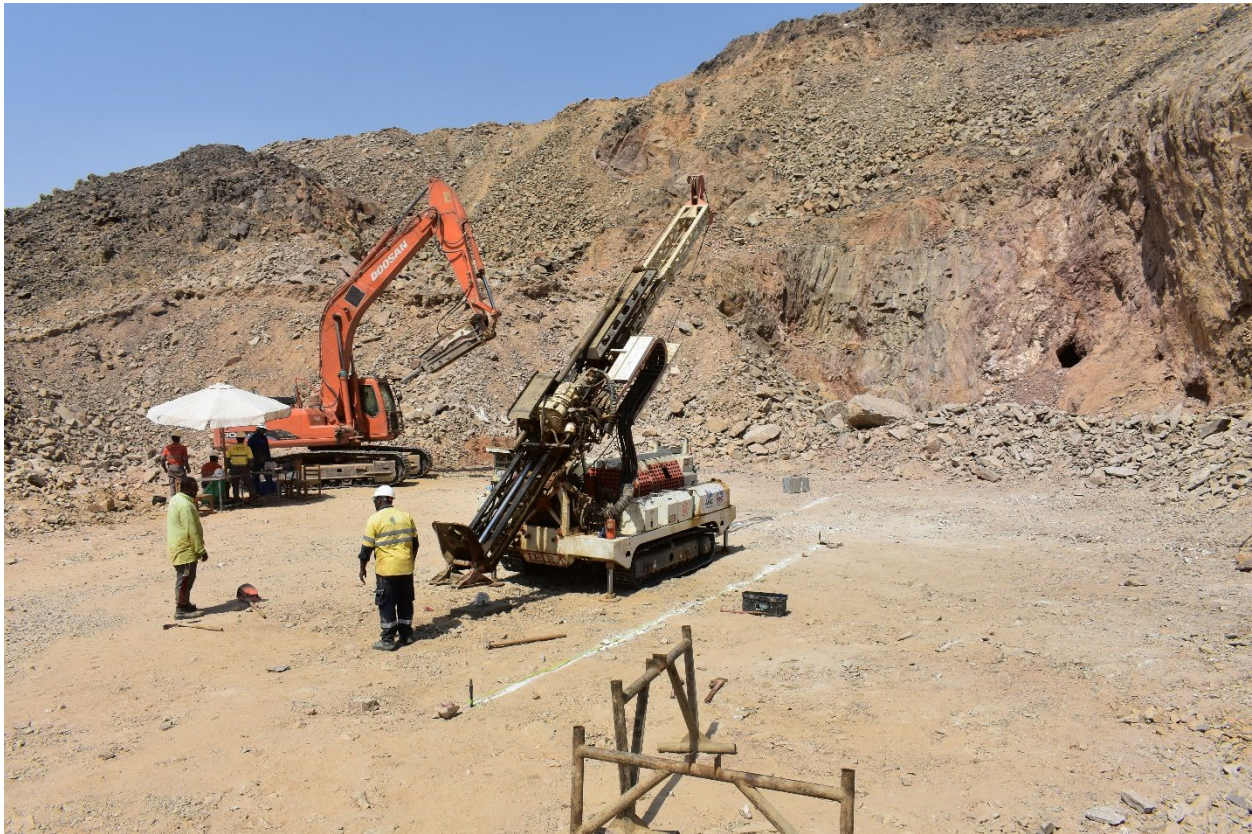
Figure 18. Set up of Diamond Drilling equipment for drill hole RMDD003.
