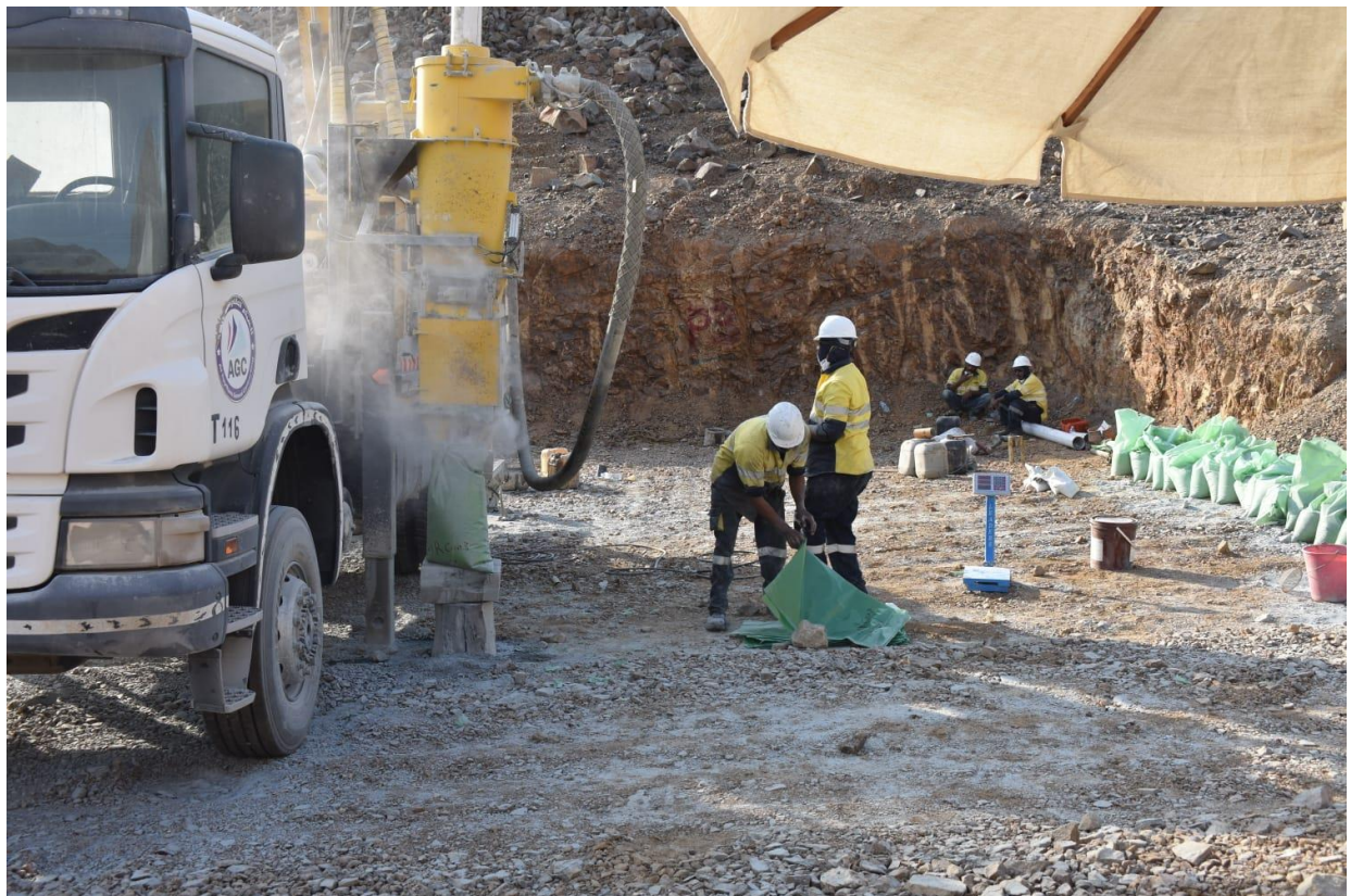
Figure 22. Site Photos from the Reverse Circulation Drilling at Romeit Occurrence
